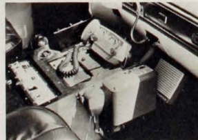
Ambulance mobile repeater radio
