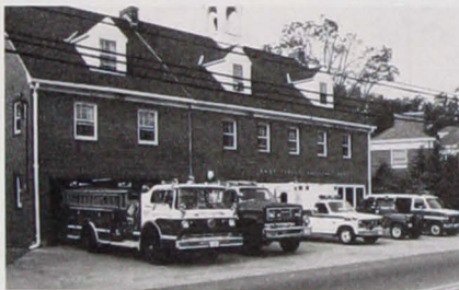
Station 4, Sandy Spring Volunteer Fire Dept. morning line-up for inspection. (Photo by George Smith)
